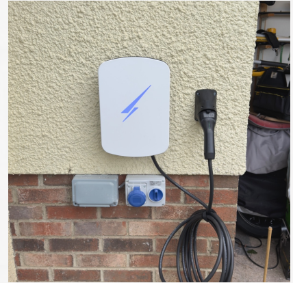
EV charger installation
